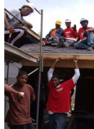
BlitzBuild 2009 with Habitat for Humanity Detroit.
