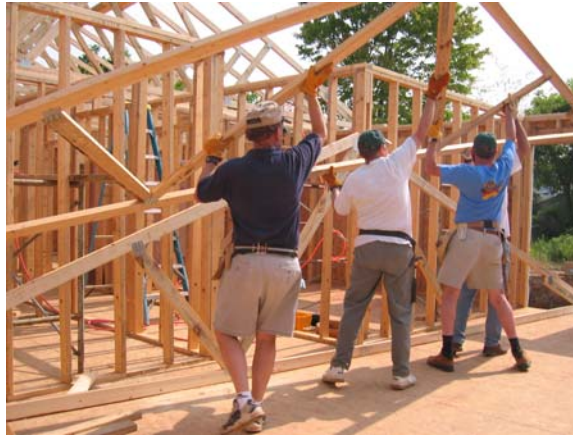
Habitat home build.
